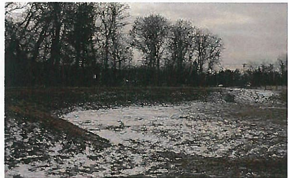
Example of Dry Extended Detention Pond
