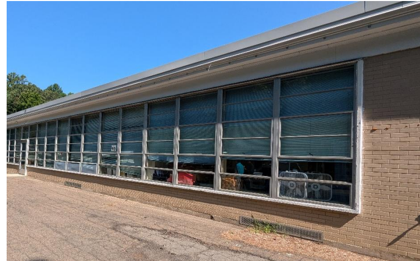
Storefront window assemblies used at pre-1996 classrooms (above)
