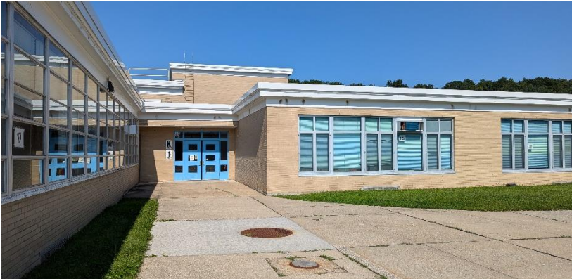
Bungay Elementary School's east elevation leading to its main entrance
